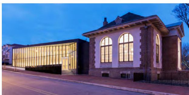
New York Public Library, Stapleton Branch, Staten Island. Example of blending new and existing construction together.
