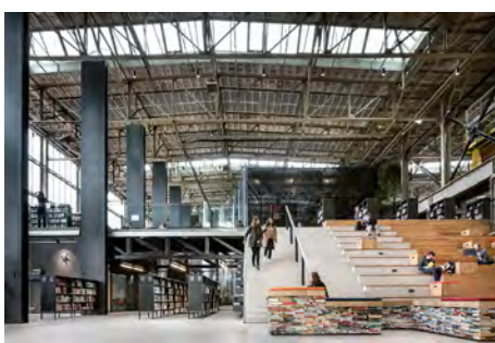
LocHal Library, Rillburn Netherlands. A former locomotive station "rebuilt" with a library inside the existing structure.
